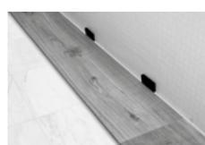
Leave a distance of 5 mm on the entire room perimeter and from every obstacle that could compromise the laying movement.
